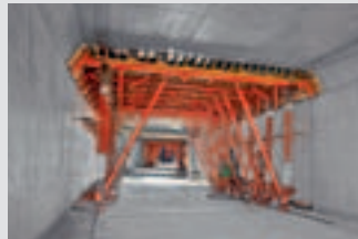
Tunnel Formwork
