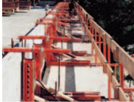
Wall Clamp 75 for fixing pre-cast parapet sections.
