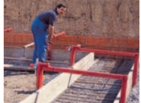
Foundations up to 90 cm wide are formed using the wall clamp 105.
