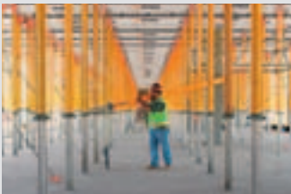
Slab Formwork
