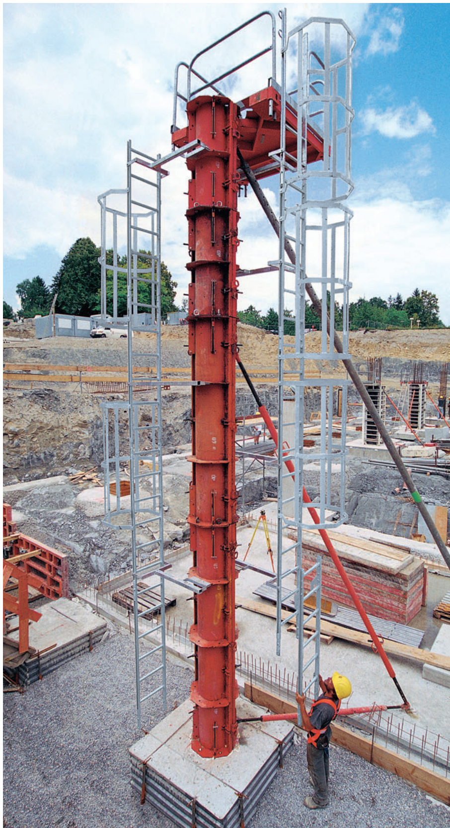
Safe working on the PERI concreting platform at all heights.
