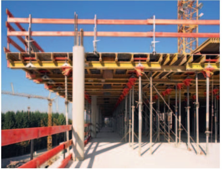
Cantilevering Table Modules VT. The anchoring chain is clearly shown here.
