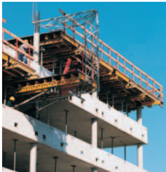
Vertical moving of PERI slab tables.
