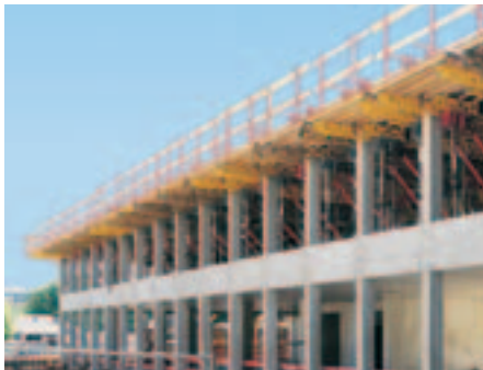
Slab edge tables with integrated safety guardrail for an administration building.
