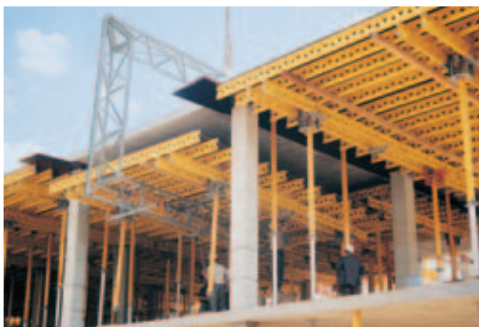
Moving of 5.40 m x 7.00 m UNIportal slab tables.
