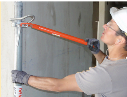
Ergonomic operations through offset wingnut spanner.
