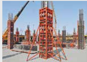
Column Formwork
