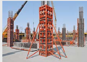
Column Formwork
