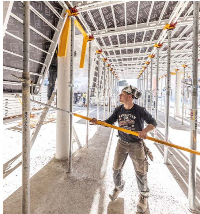
With the shuttering aid you can safely form room heights of at least 3.80 m.
