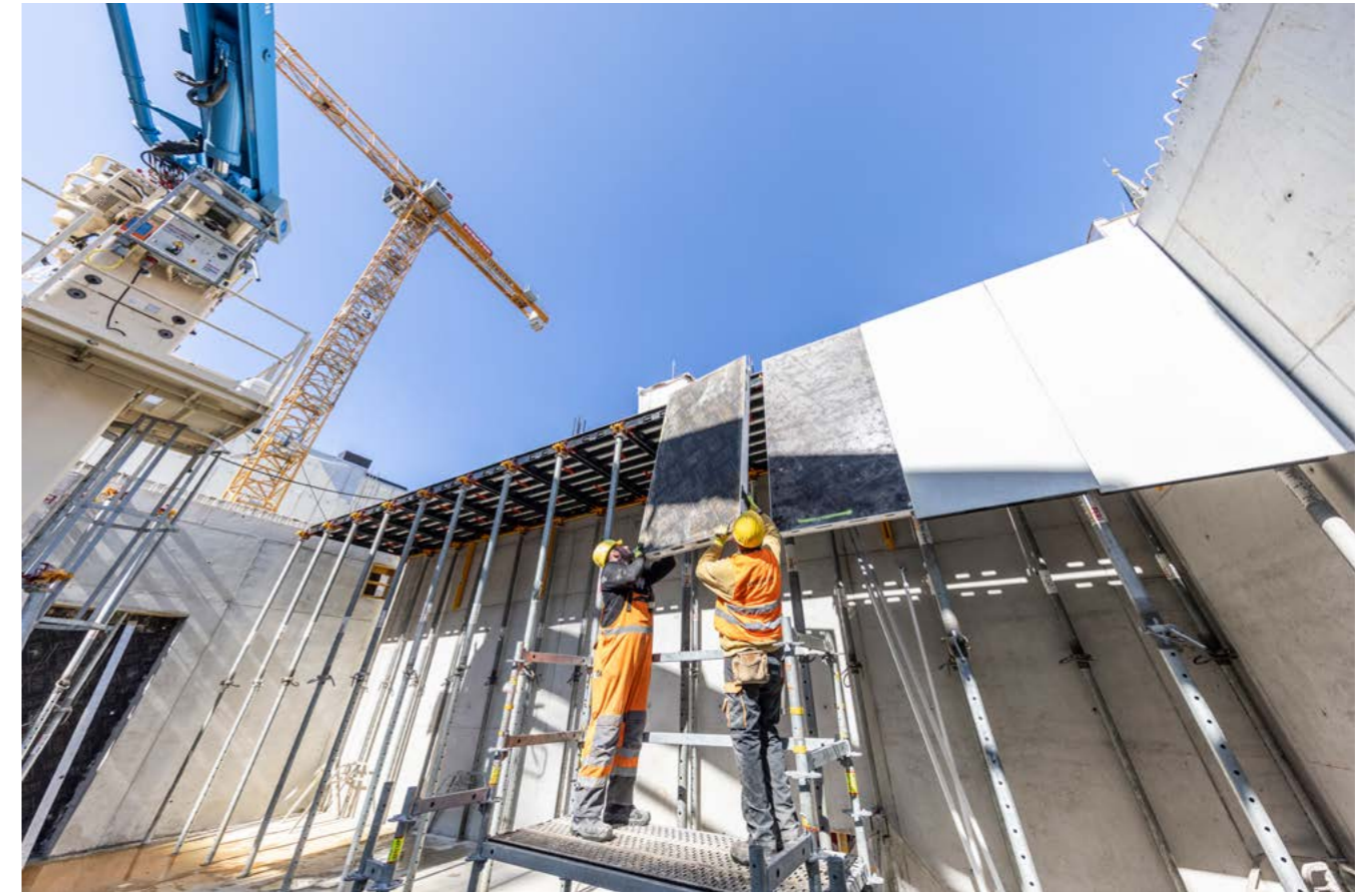
Even high slabs exceeding 3.80 m can be formed from the level below with PERI system components. The compatibility of the aluminium and polymer components enables you to optimally adapt them to your construction site requirements.
